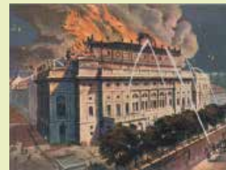
The Fire at the National Theatre (12 August 1881).
