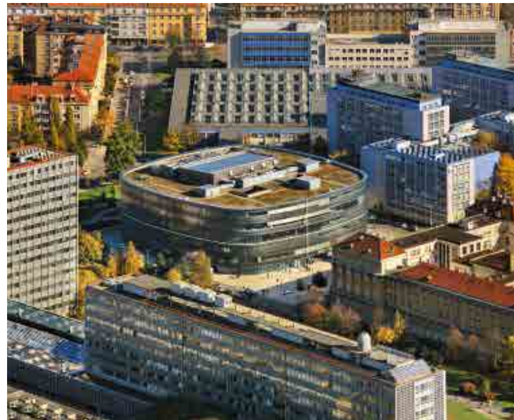
National Technical Library in Dejvice.
