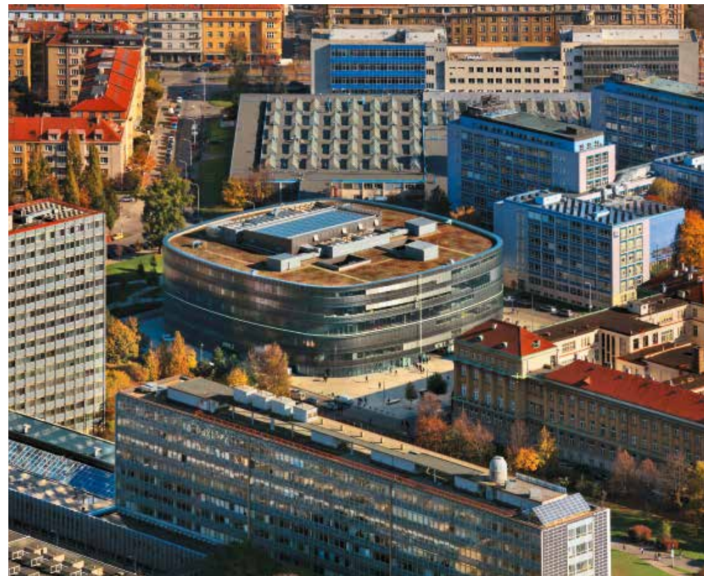
National Technical Library in Dejvice.
