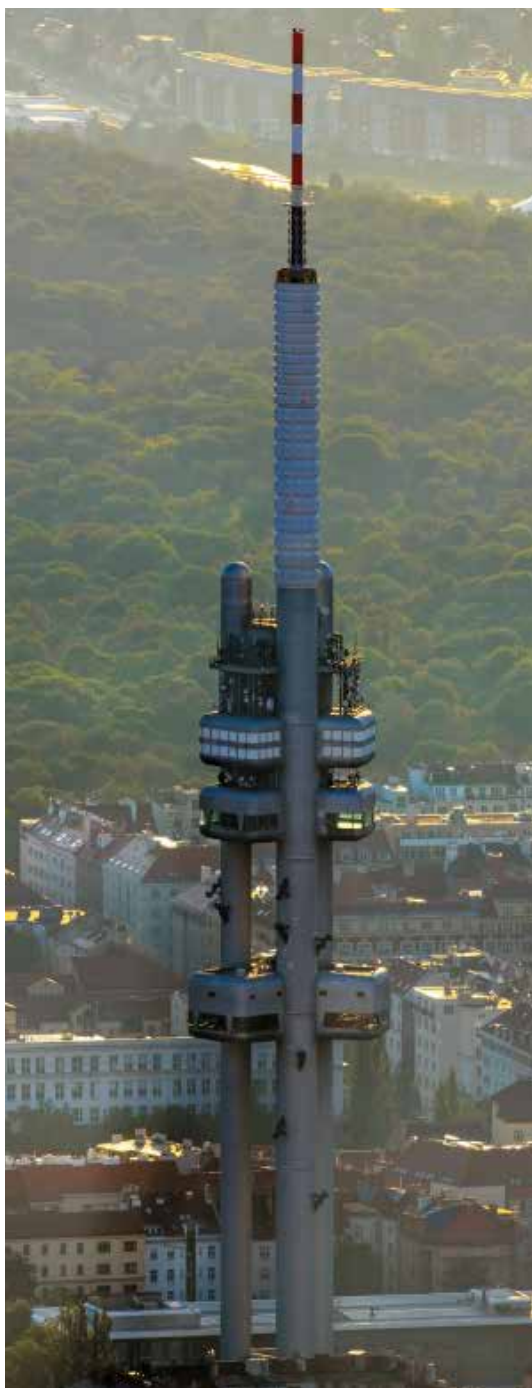
The Žižkov TV Tower is the tallest structure in Prague (216 m).
