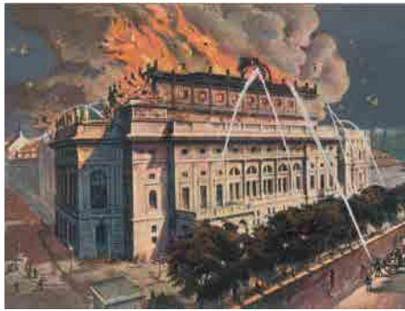
The Fire at the National Theatre (12 August 1881).
